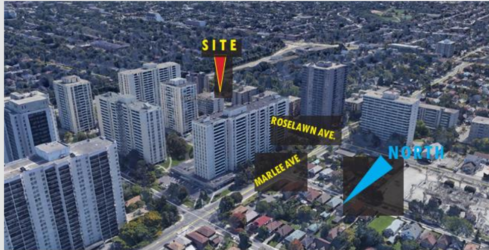
A-View Looking South-East
