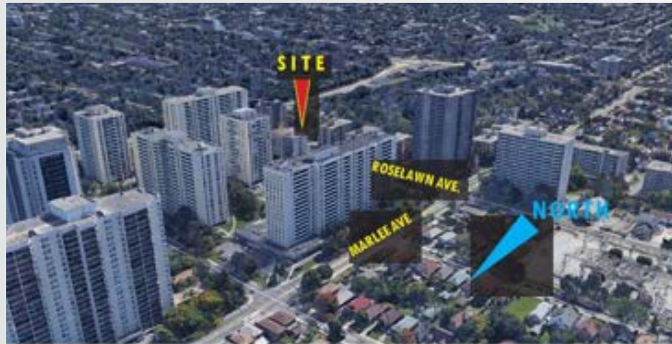
A-View Looking South-East
